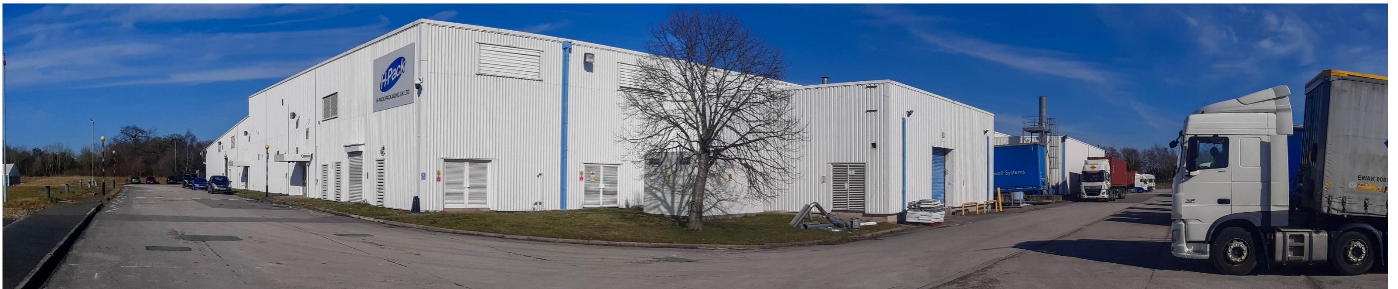
Stitched panoramic photograph northeast from the existing shared yard area, showing the H-pack buildings, with the application site to the left.
