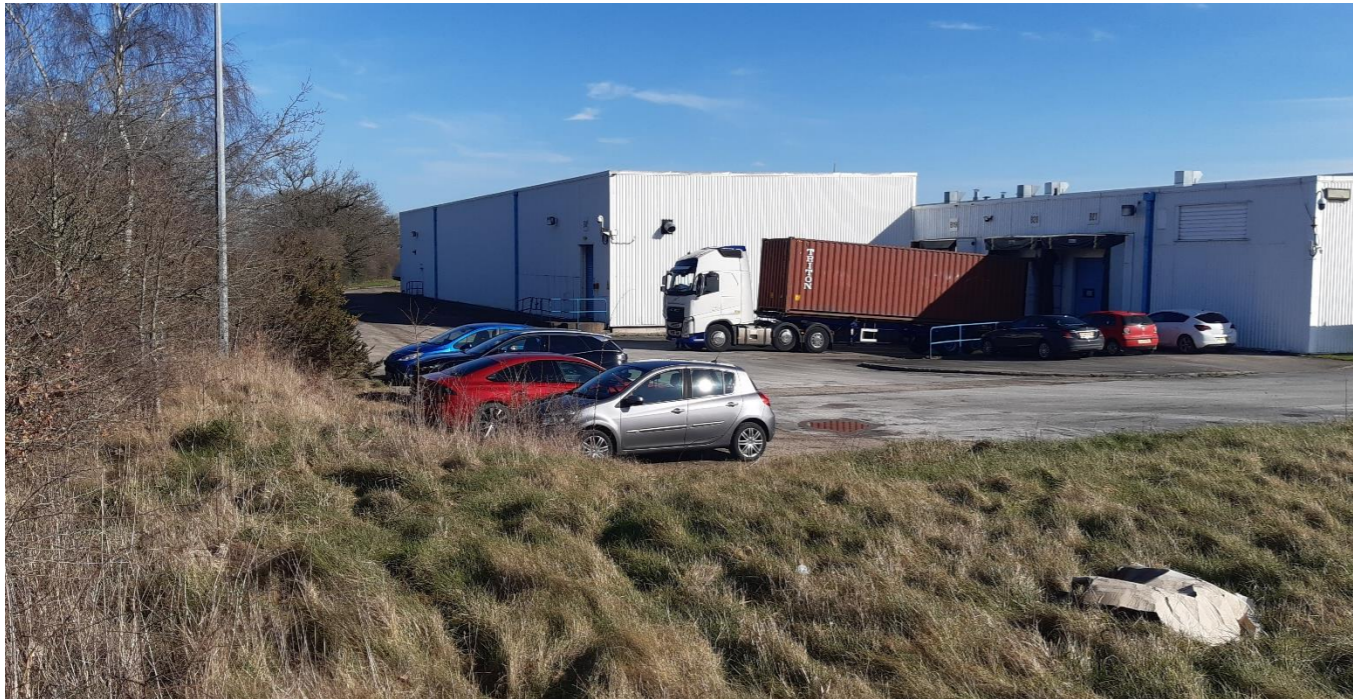
Existing facility, viewed from the northern boundary.
