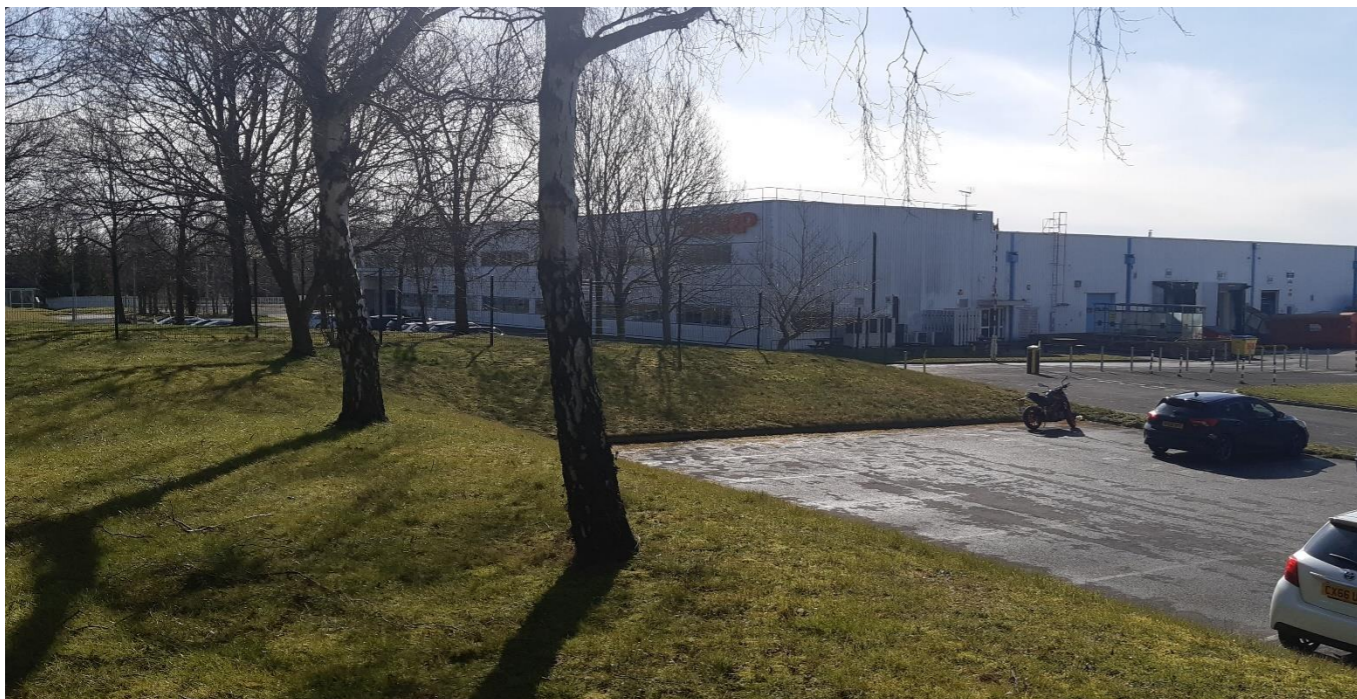
View south across eastern boundary towards H-Pack's existing facility
