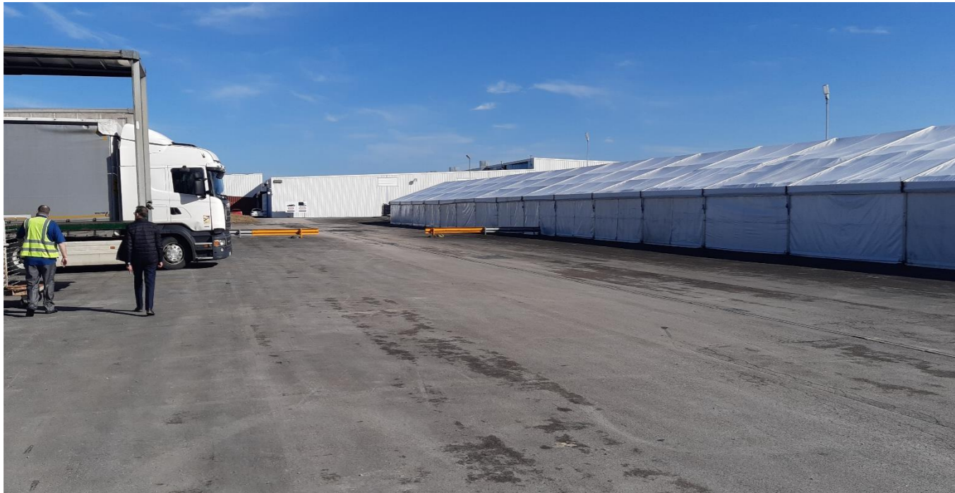
Existing temporary structures on the development plot on the hardstanding areas
