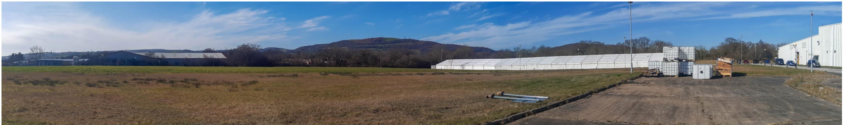
Stitched panoramic photograph northeast from the proposed yard area, across application site, showing the existing temporary structures centrally, existing facilities to the right, and established landscaping beyond.
