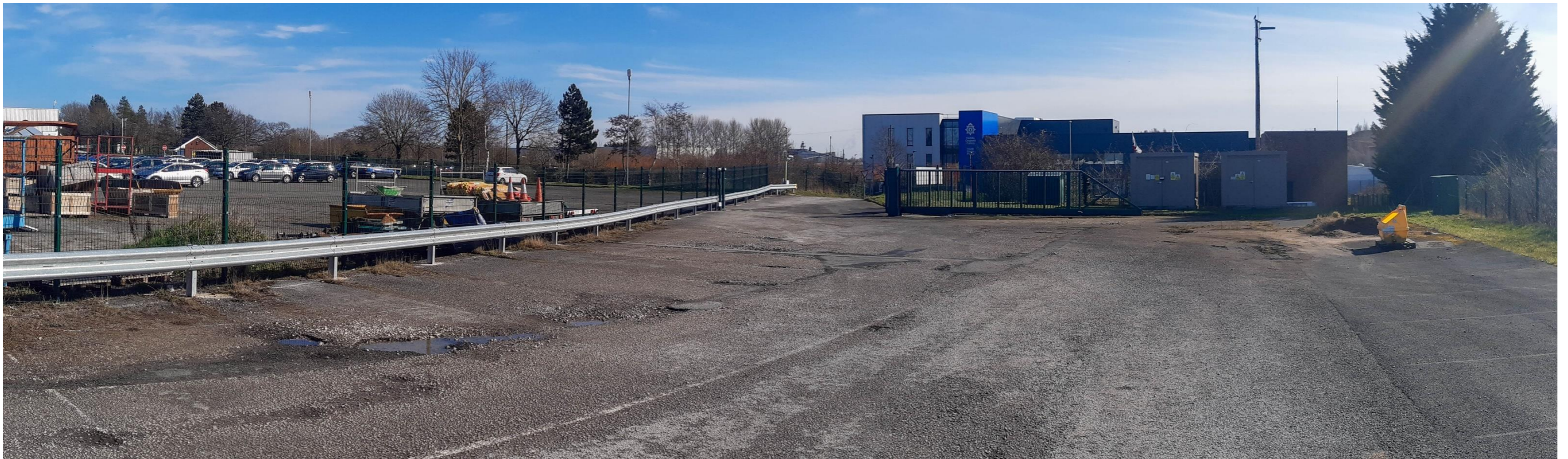
Stitched panoramic photograph taken at the existing vehicle entrance looking southwards towards Davy Way and the North Wales Police building
