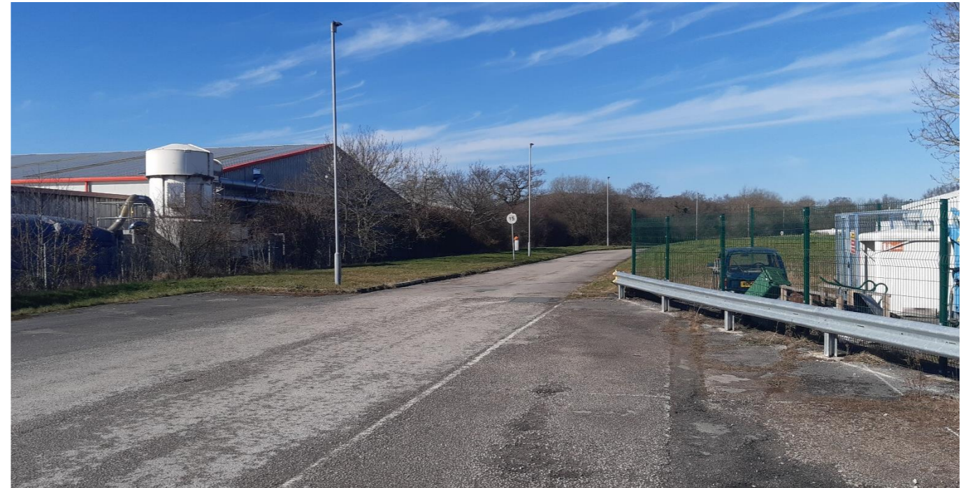
Existing internal vehicle route with Marlin buildings on the right
