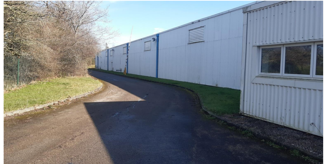
View eastwards along the northern boundary showing the access road leading to H-Pack's surface level car park
