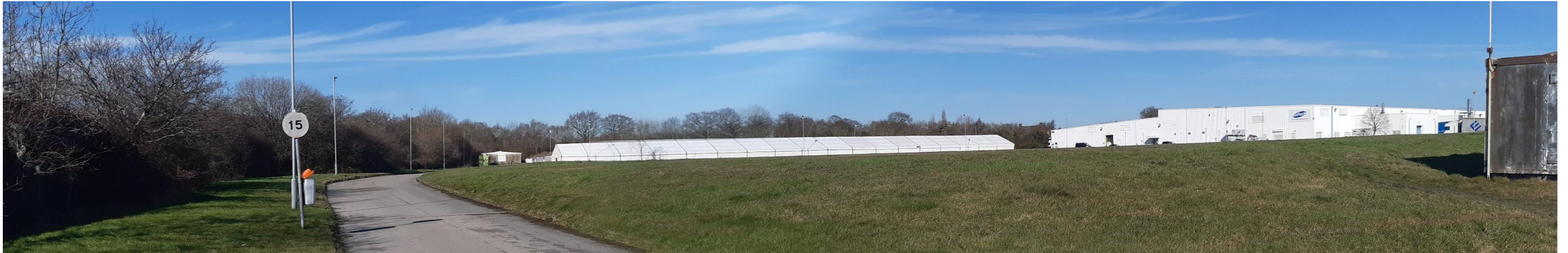
Stitched panoramic photograph northwest from the vehicle access across application site, showing the existing temporary structures centrally, existing facilities to the right, and established perimeter landscaping to the left.
