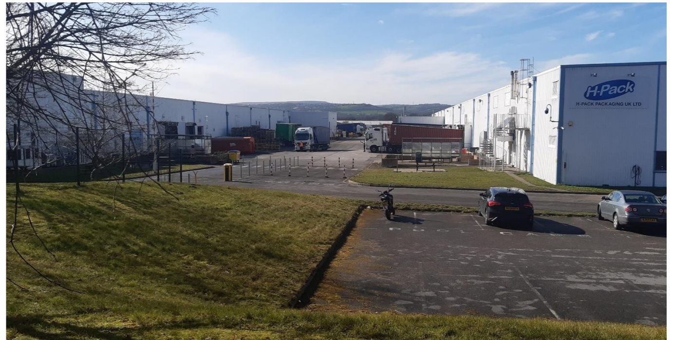
View southwest towards the shared service area.
