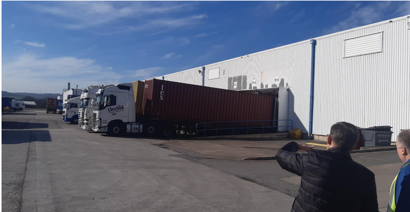
View westwards along the south-eastern elevation of the existing facility showing dock levellers accessed via the shared service yard
