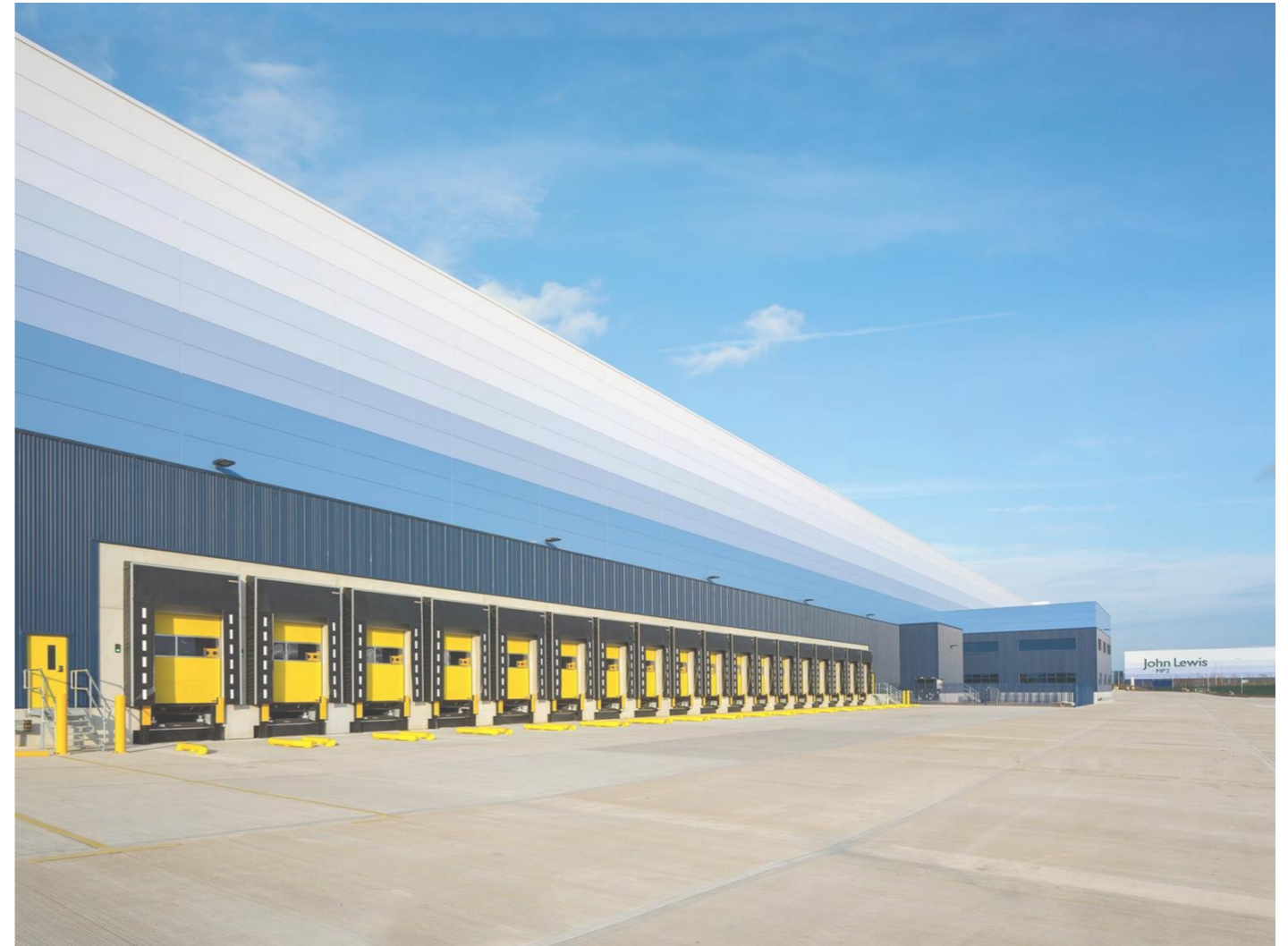
Industrial development at Magna Park, Milton Keynes, where a graded cladding treatments (blue-to-white in this example) have been implemented to soften the scale and massing
