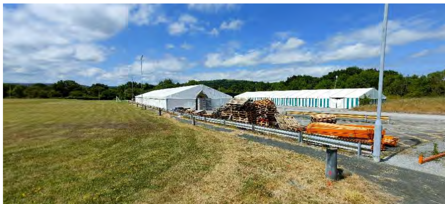
20. Eastern part of Development Site, football pitch to the left, access road and temporary storage units to the right.
