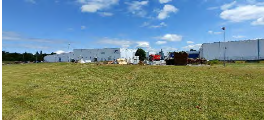
16. H-Pack warehouse to the left and SHARP warehouse to the right along the eastern Development Site boundary.
