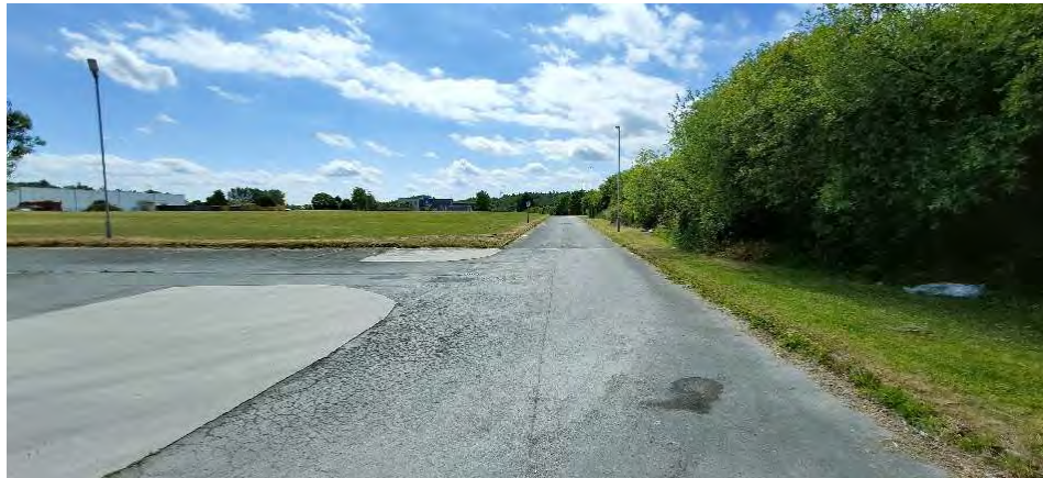
22. Access road west of the Site, view towards the south.
