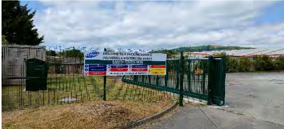
7. Second entrance gate, electrical substation units to the left.
