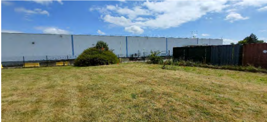
13. View towards the south-eastern corner of the Development Site, SHARP warehouse behind.
