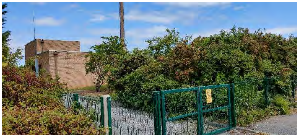
3. Electrical Substation in the southern tip of the Site.
