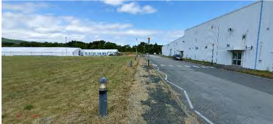
19. Eastern boundary of Development Site, view towards the north and H-pack warehouse to the right.
