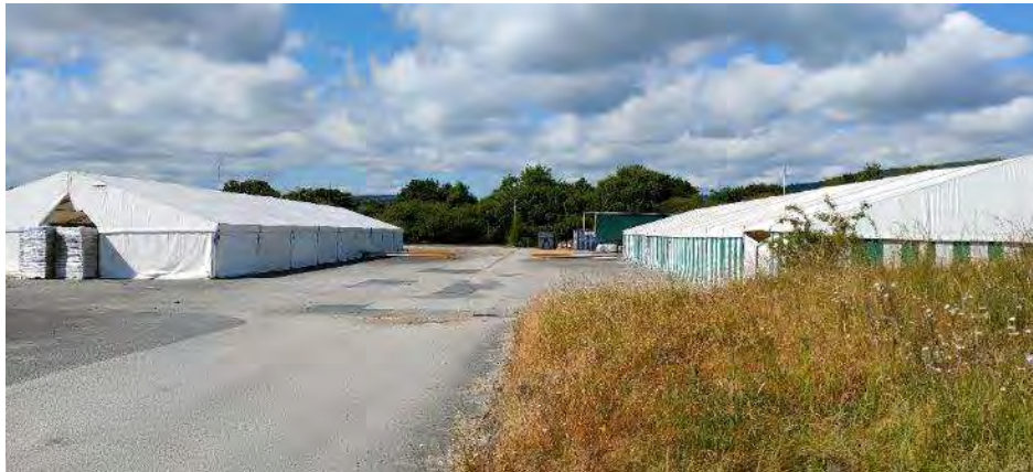
28. Access road to the north with temporary storage units.
