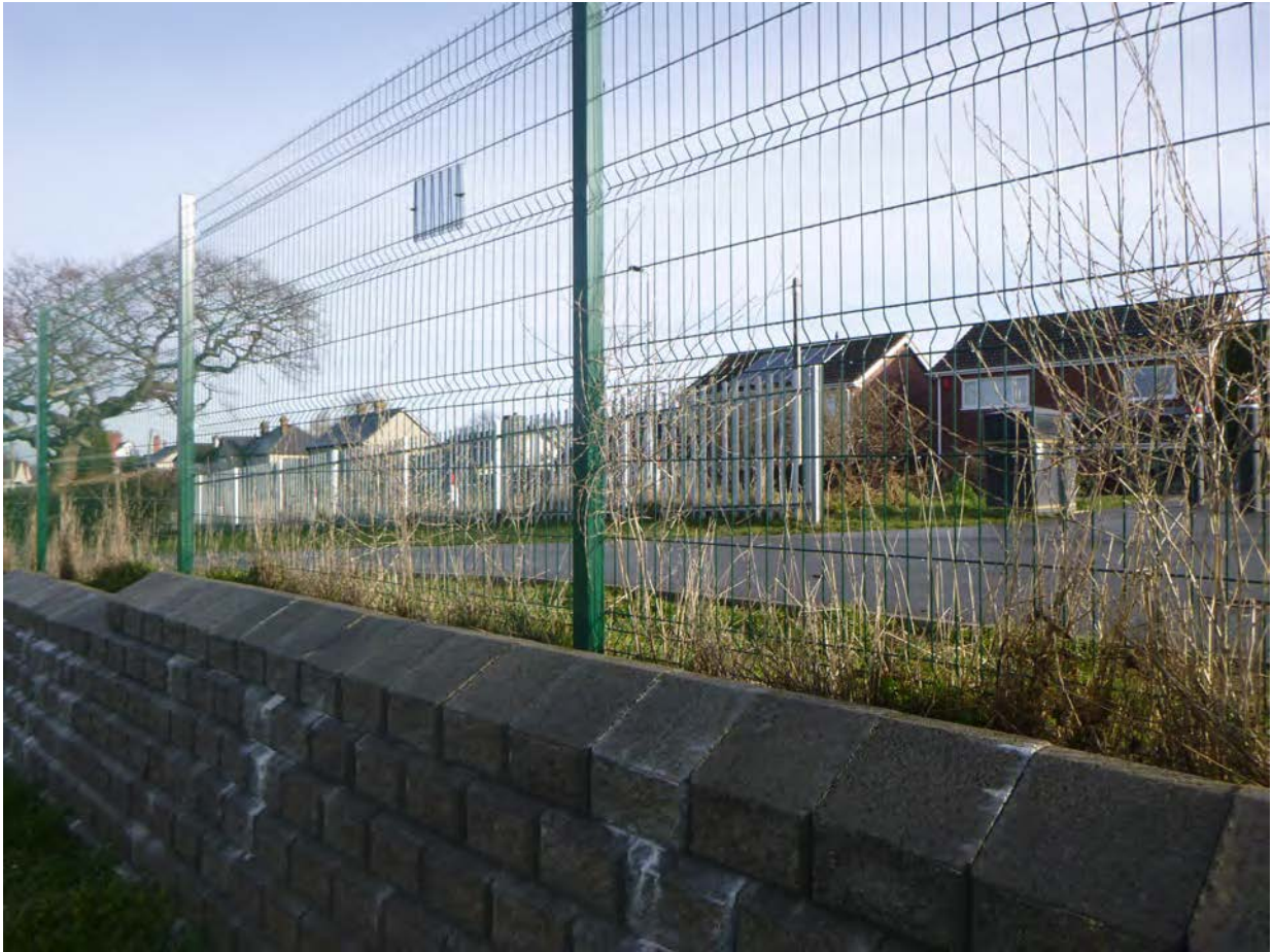
Plate 10. View from E of site looking N
