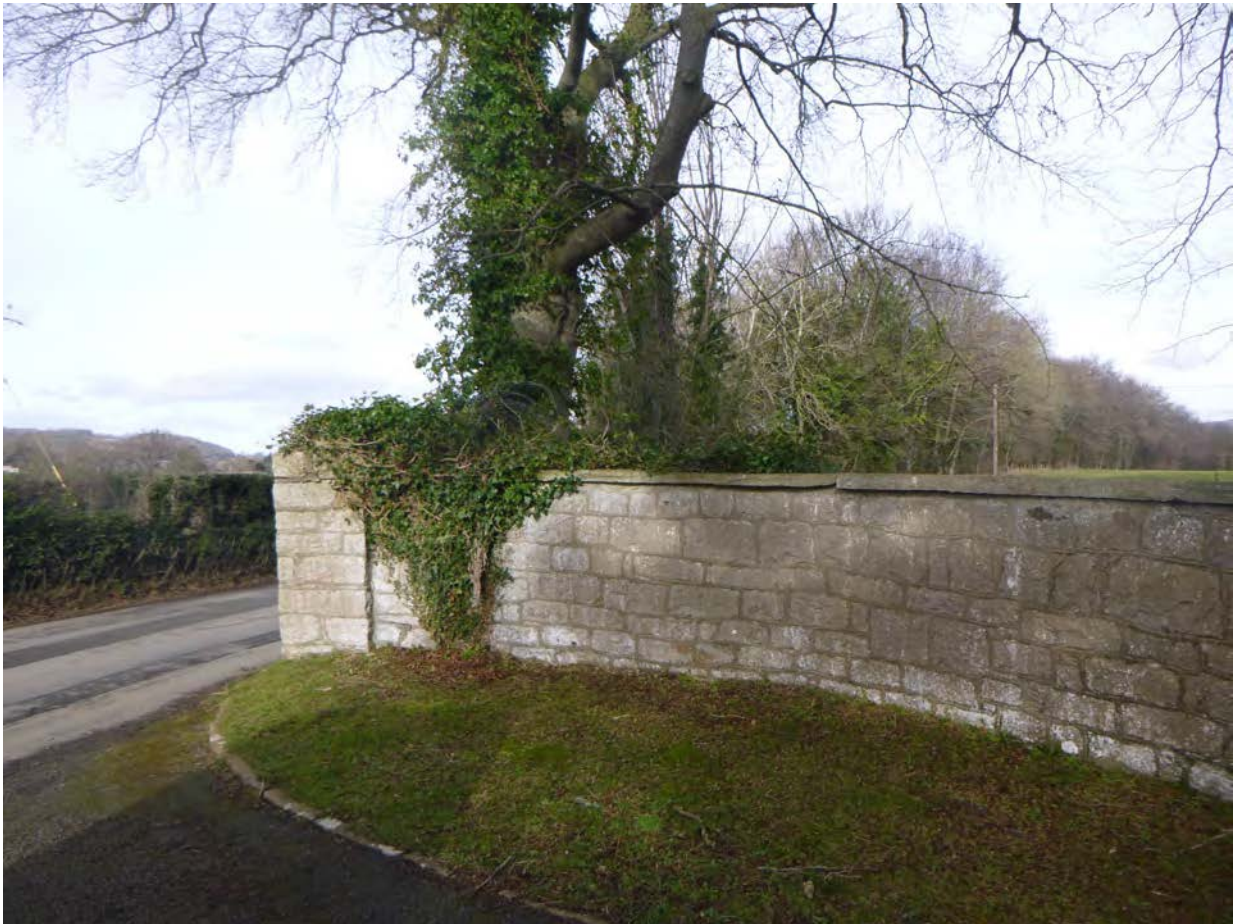
Plate 32. Parish Church of St Marcella toward site
