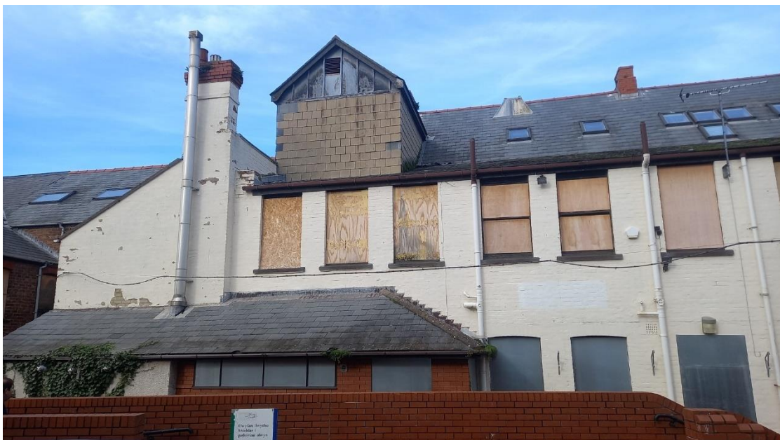
Fig. 9 Site Image, rear elevation
