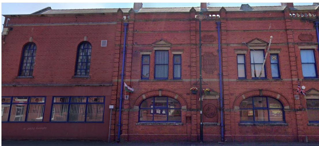
Fig. 5 Elevation fronting Nant Hall Road, 1903 Date Stamp
