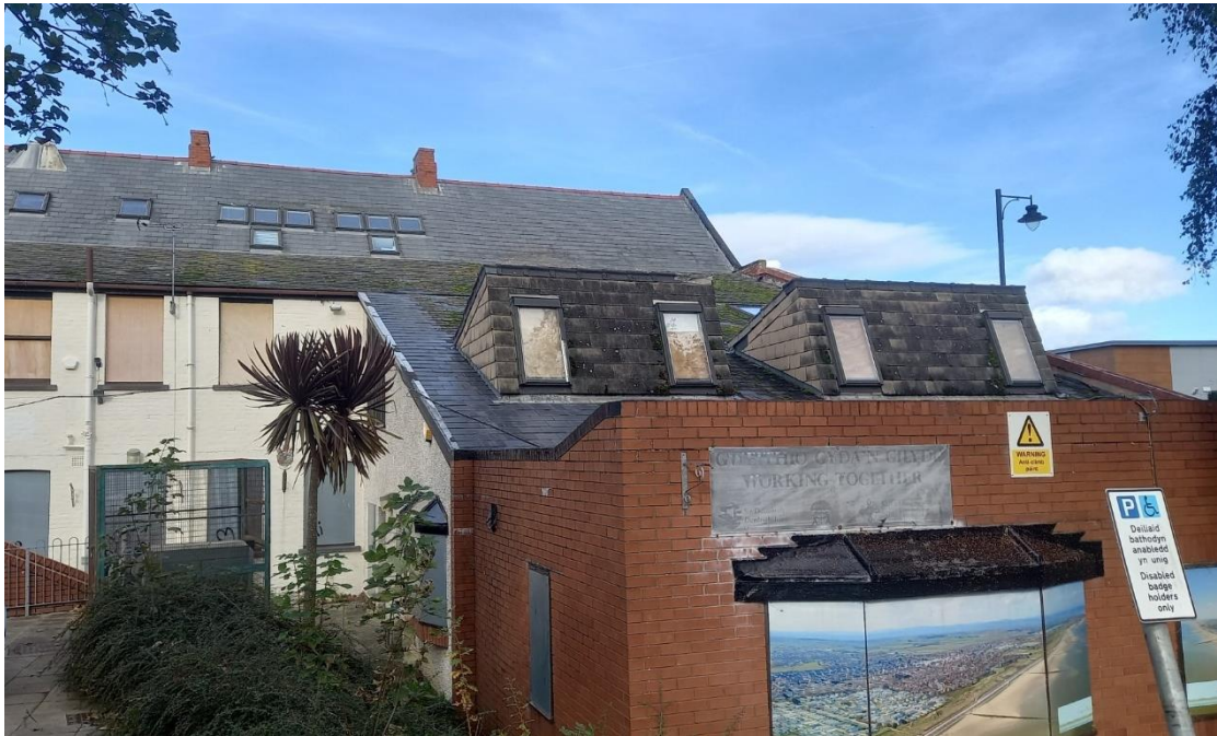
Fig. 8 Site Image, rear elevation
