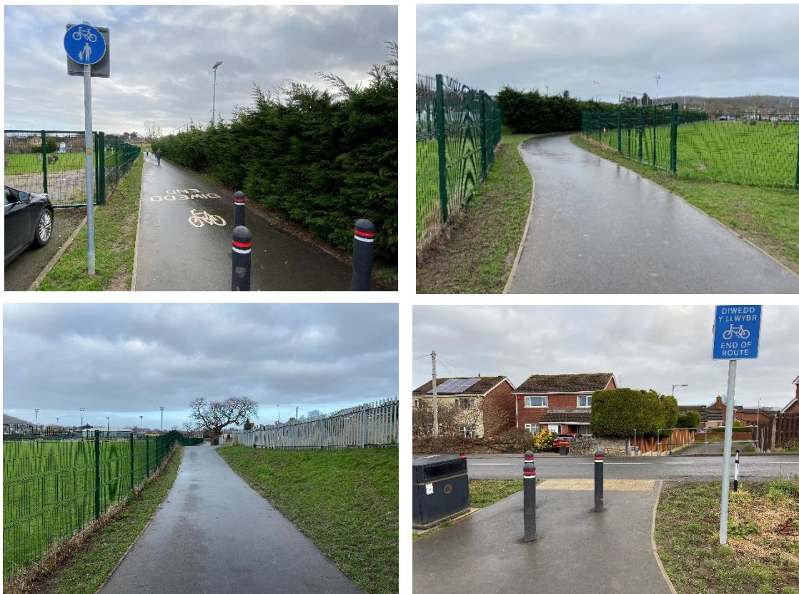
Figure 4.2 – Existing Active Travel Route (Site Photographs)
