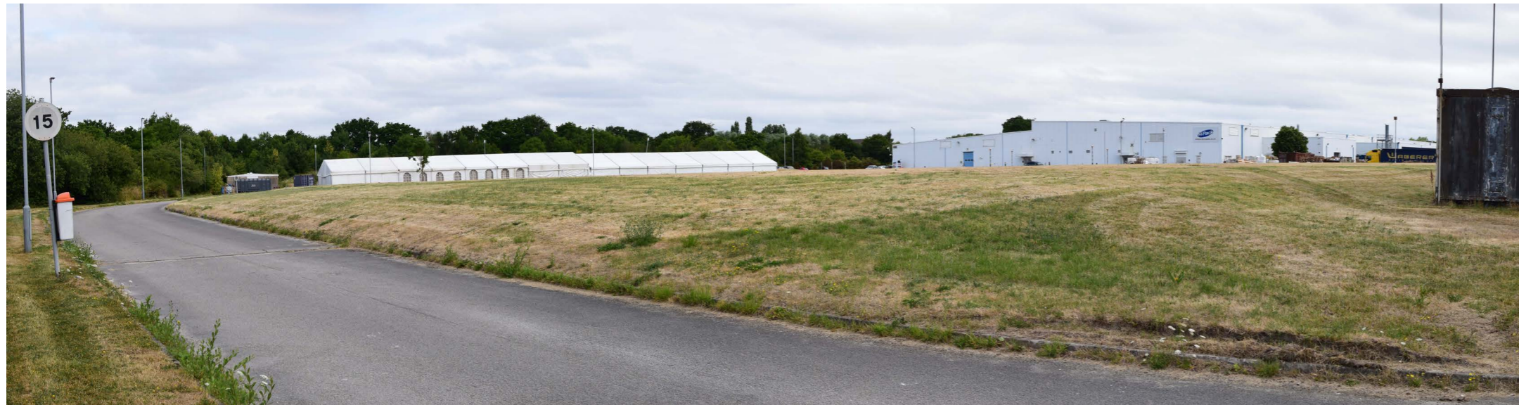
Site Photograph B - View looking north across the site
